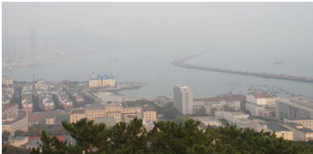
Photo 14: The uncompleted Dalian Xinghai Bay Cross-sea Bridge (Pulandian Bay Bridge). It is said to be the biggest continuous beam sea-crossing bridge in Northeast China and replaces the congested coastal road.
